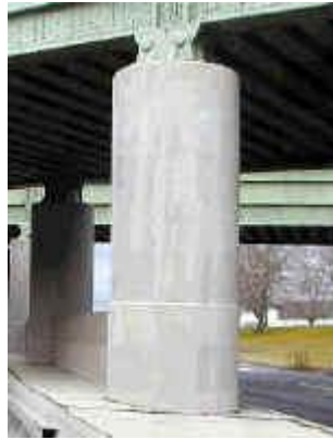
Filler material used to restore shape
