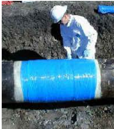
Stricture Banding™ is used to compress and consolidate the composite
