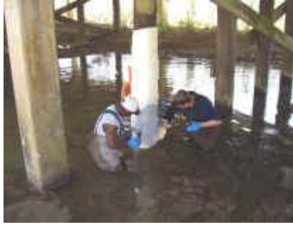
Final Layer of BP-4 Coating
