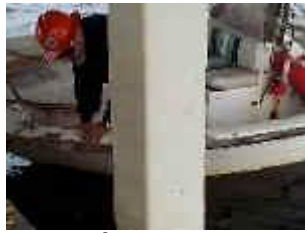
Aquawrap® Installation Complete
