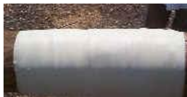
Final Coat of Aquawrap ® G-03
