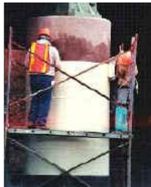
Aquawrap® G-05 Installation
