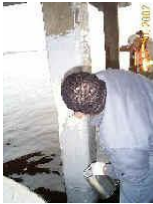
Final protective coating applied
