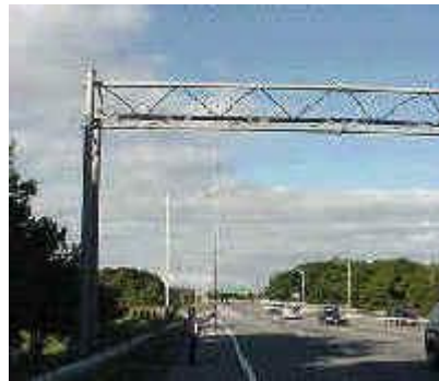
Typical Sign Structure
